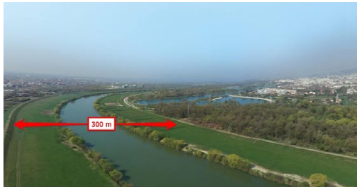
Figure 2. Defensive embankments along the river Sava through the urban area
